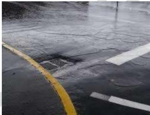
Figure 1: Stormwater draining from a parking lot
